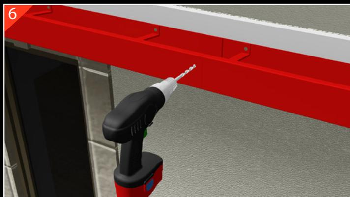
Next drill out the holes marked with indentations on the female end of the gutter (two in the front and two in the base). Note the holes should be positioned between the two rows of butyl tape, therefore the silicone will secondary seal when the rivets are installed as below.
