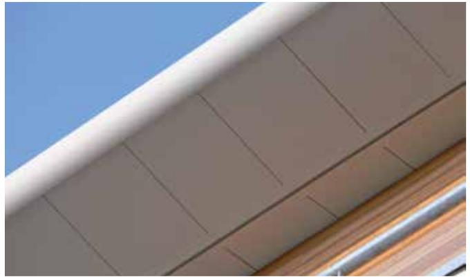
ALUMINIUM BULLNOSE FASCIA & ARROWHEAD SOFFIT PLANKS
