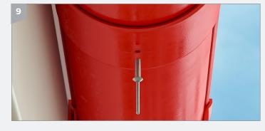
Drill through the existing 3mm hole in the bottom of the joining strap. Then, to secure the joining of lengths insert 4.8mm Ali sealed rivet (GM10) through the drilled hole. Use a rivet gun (GM67) to fix the rivet securely.
