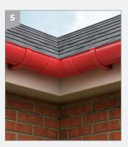
Support angles by fixing fascia brackets a maximum of 150mm from each side.
