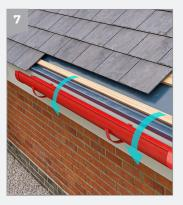
Place the gutter into the fascia bracket by rolling into position, then snap the gutter fully into the fascia brackets.
