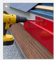
Level the first length and fix directly through the crossbrace at the back of the gutter with 38 x 5 stainless steel screws (GM1).
