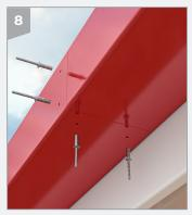
To secure the joining of lengths insert 4.8mm
