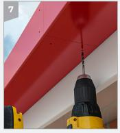
Drill the 4 holes marked with indentations in the first gutter length (female end), two located at the base of the gutter and two in the front.
