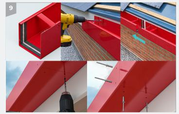
Repeat stages 3, 4, 6, 7 and 8 and joint the gutter length to the one previously fixed.
