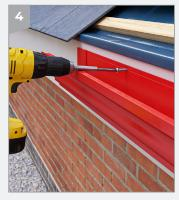
Level the first length and fix directly through the back of the gutter with 38 x 5 stainless steel screws (GM1).
