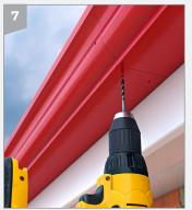
Drill the 3 holes marked with indentations in the first gutter length (female end), two located at the base of the gutter and one in the front.
