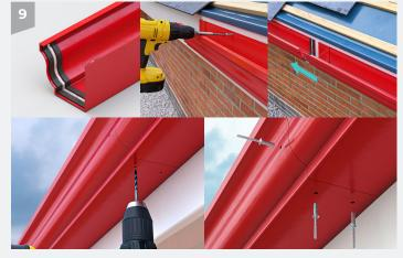
Repeat stages 3, 5, 6, 7 and 8 and joint the gutter length to the one previously fixed.
