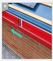
Repeat step 2 then firmly place the male end of the gutter onto the siliconed joint. Ensure the top of the gutters are fully aligned. Screw to secure as explained in step 3.
