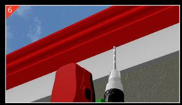
Next drill out the holes marked with indentations on the female end of the gutter (one in the front and two in the base). Note the holes should be positioned between the two rows of butyl tape, therefore the silicone will secondary seal when the rivets are installed as below.
