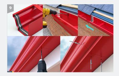
Repeat stages 2, 3, 5, 6, and 7 and joint the gutter length to the one previously fixed.
