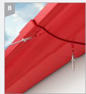
To secure the joining of lengths insert 4.8mm Ali sealed rivets (GM10) through the drilled holes. Use a rivet gun (GM67) to fix the rivets securely.
