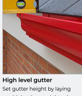
Set gutter height by laying a spirit level or straight edge level against the lowest point of the roof tile to determine the position of the bracket.
