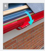
Repeat step 2 then firmly place the male end of the gutter onto the siliconed joint. Ensure the top of the gutters are fully aligned. Screw to secure as explained in step 3.
