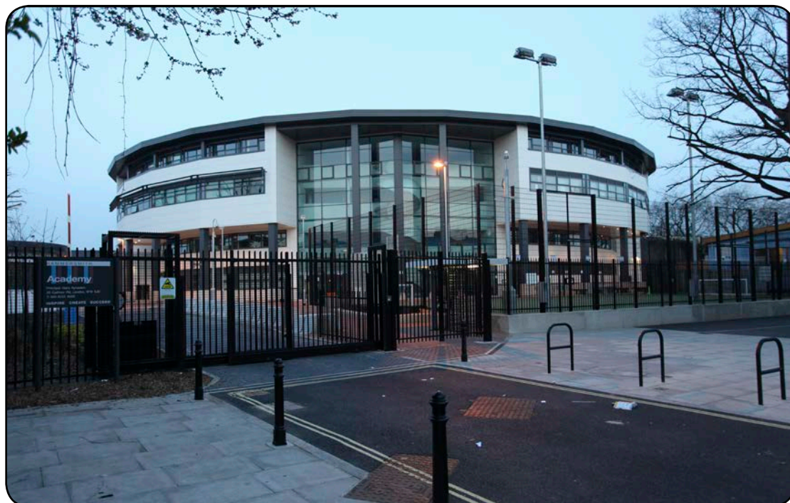
Aluminium Fascias, Tapered Arrow Head Soffits, Column Casings and Copings.
