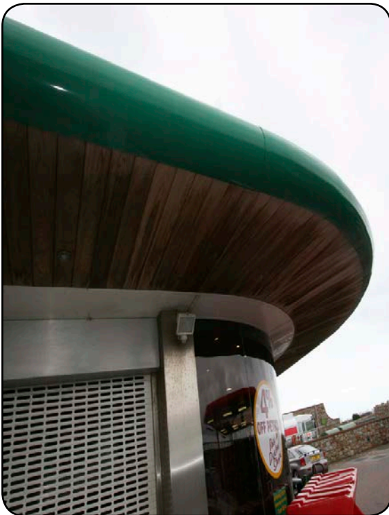
True Curve Bullnose Fascia junction to Straight Bullnose.
