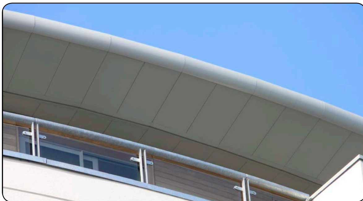
Bullnose Fascia Segmented with Tapered Arrowhead Soffits.
