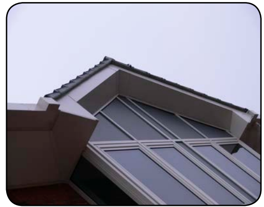
Duo Fascias and Soffits with Boxing at Gable Junction.
